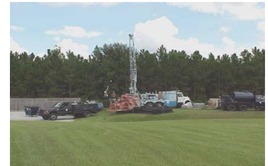
Monitor Well Construction – Pasco County
